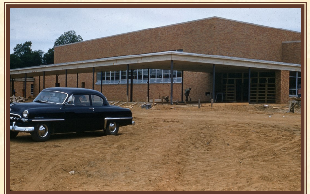
Wantagh High School Under Construction
